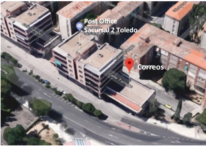
Aerial view of Toledo, Spain post office .
